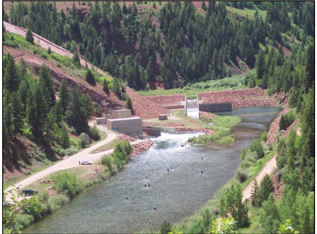
Ruedi Reservoir in Pitkin and Eagle counties, located on the Fryingpan River, filled and spilled this past spring. Pictured are the hydro power plant on the left and the dam spillway on the right. Anglers can be seen enjoying casting for fish in the dam's tail waters.
