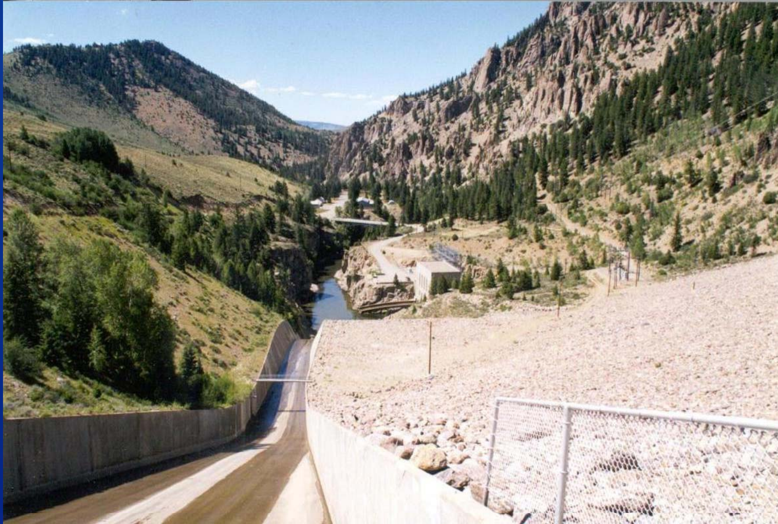
Green Mountain Dam and Powerplant on the Lower Blue
