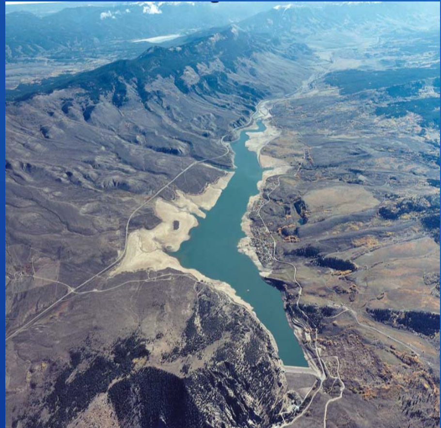
Green Mountain Reservoir in late summer 2003
