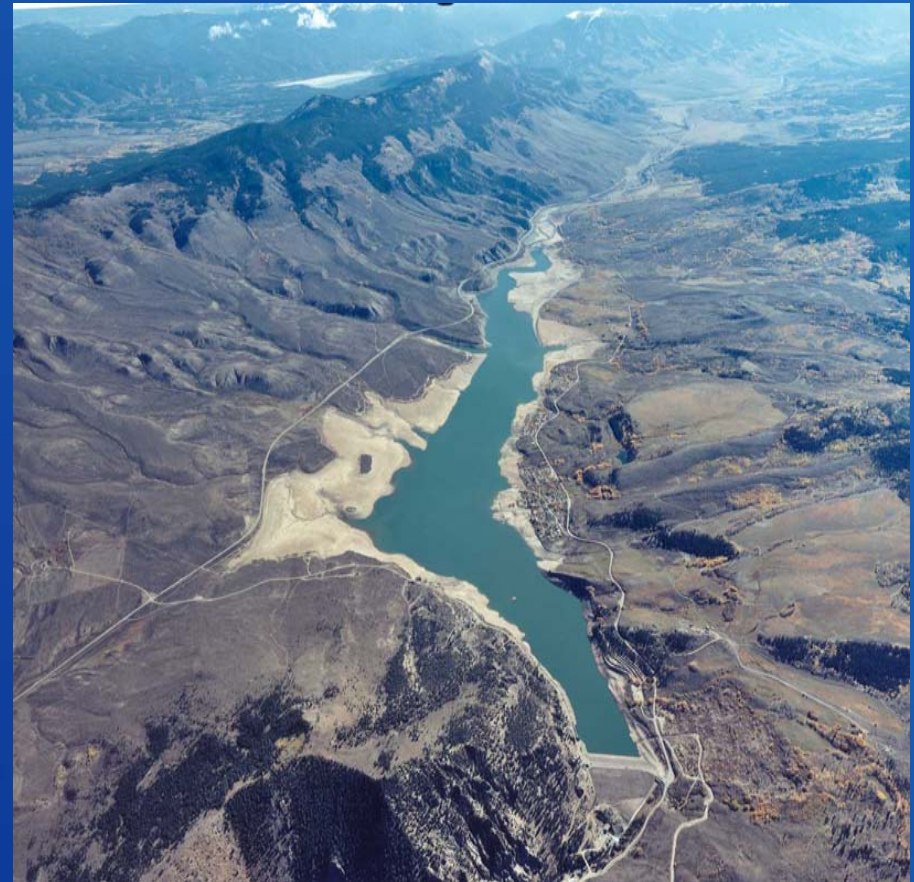
Green Mountain Reservoir in late summer 2003
